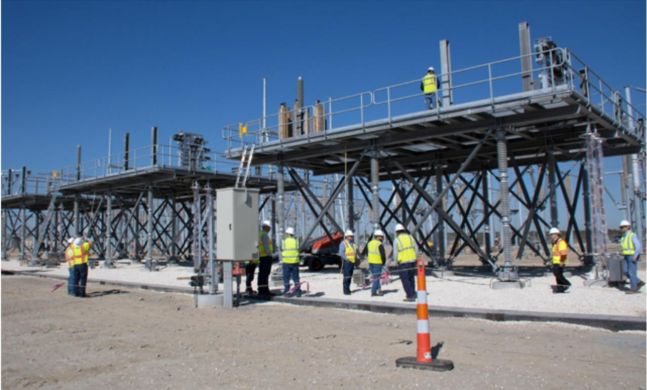
ETT also invested some \$16 million in series compensation equipment at Del Sol and Cenizo (photo right during construction) stations to maintain acceptable voltage levels across long distances, reduce impedance on the lines, cut system losses and ensure reliability. General Electric, the manufacturer, installed the equipment that went into service in May
